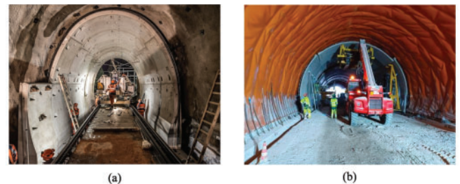
Figure 15. (a) Precast segment installation in the Glatscheras tunnel 53 and (b) precast predalle positioning in the Colle Marino tunnel 6
