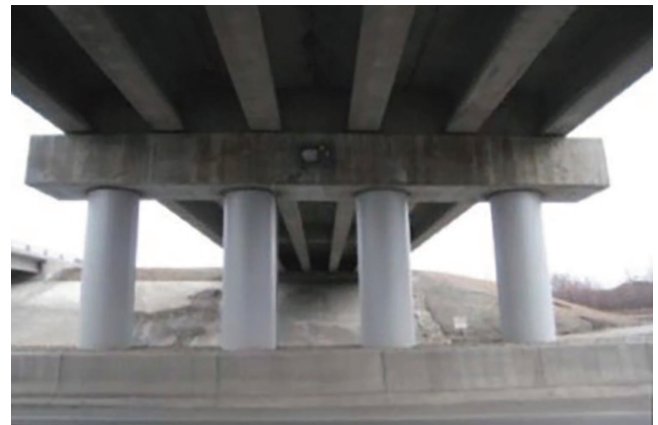
Figure 1. Example of an RCFST multicolumn bent used in the O'Malley Bridge, AK
