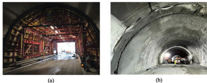
Figure 16. (a) Modified shuttering used for T3 tunnel rehabilitation 54 and (b) shotcreting of the Manfreida tunnel 6
