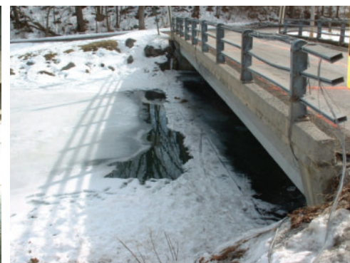
Melted ice on day of testing
