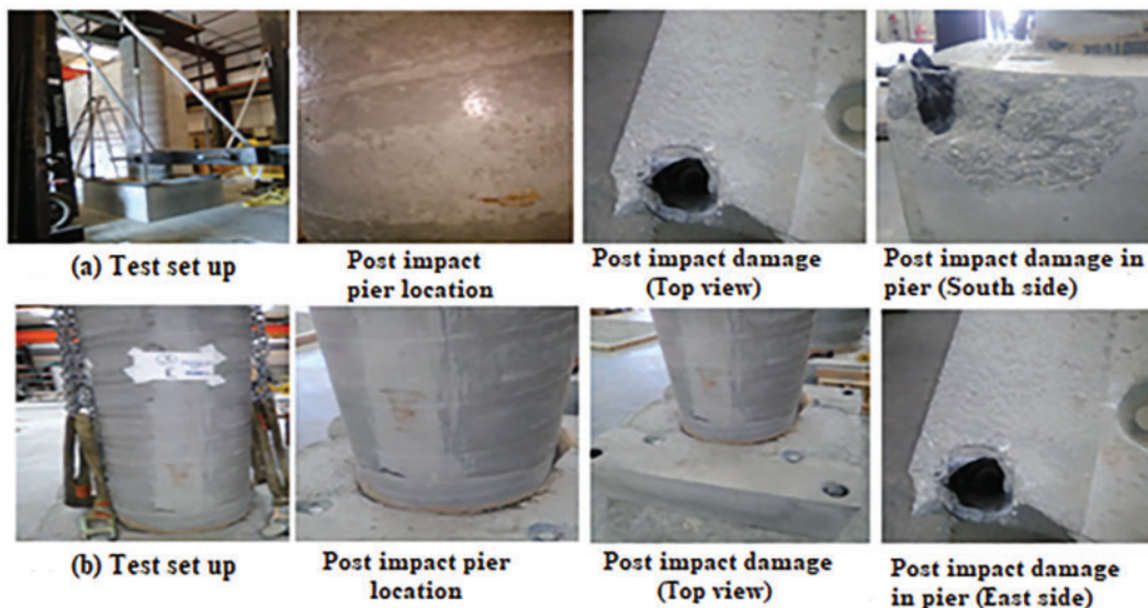
Figure 9. Pre-impact test setup and post-impacted pier damage for (a) P1 and (b) P2
