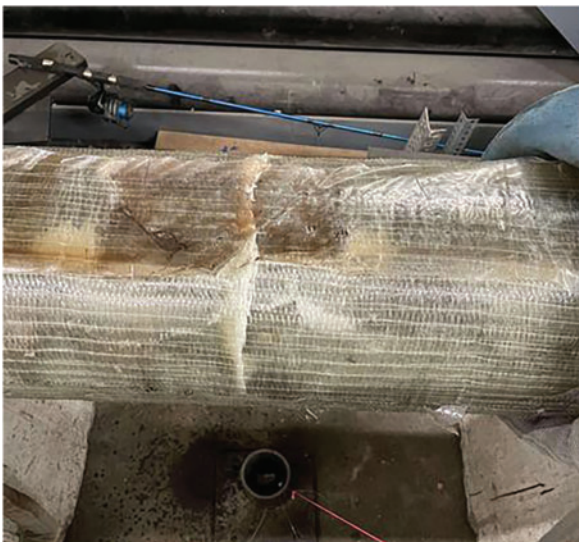
Figure 27. Compressive failure of fabric
