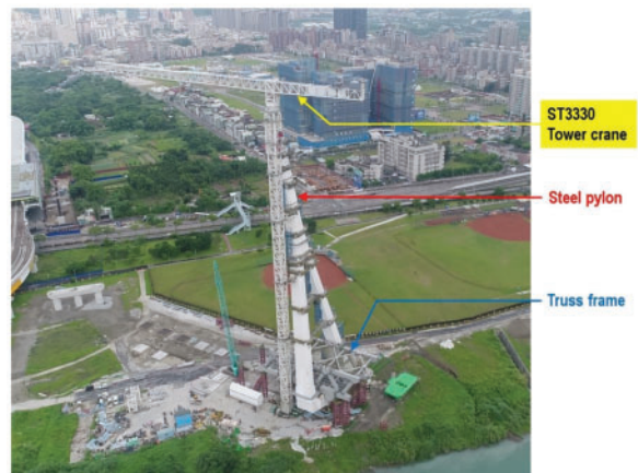
Figure 6. Photograph of the ST3330 tower crane
