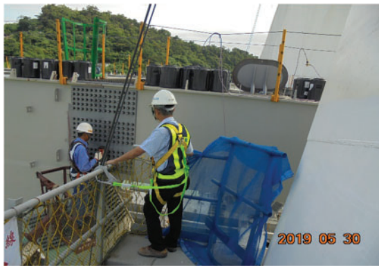
Figure 10. The responsible engineer supervising the bolt penetration of the truss-frame beams 11
