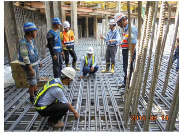
Figure 14. Inspection of the foundation by the QC engineers. QC, quality control
