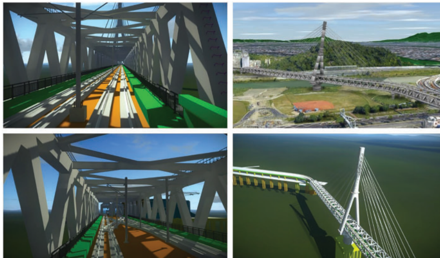
Figure 23. BIM-generated images of the AHB and the appearances of the steel truss-frame. AHB, Anhsin Bridge; BIM, building information modeling
