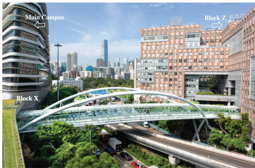
Figure 1. Bird's-eye view of the footbridge
