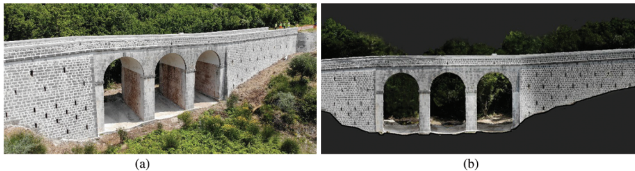
Figure 2. Example of the survey of external geometry: (a) the Bridge on SP9 in Caserta Province and (b) point cloud elaboration based on UAV photogrammetry
