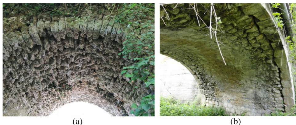
Figure 1. Examples of damage on masonry arch bridges: (a) loss of mortar joints and bricks, and (b) longitudinal crack at the arch intrados
