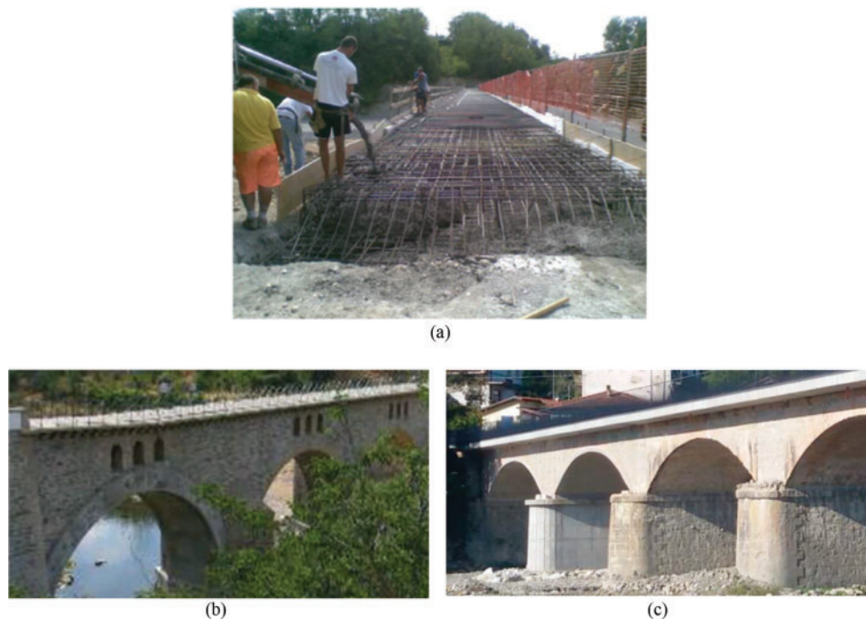
Figure 11. Examples of traditional strengthening techniques: (a) reinforcement of half-slab on the Borbera bridge; 91,112 (b) arch reinforcement with shotcrete on the Remondes Bridge; 5 and (c) rehabilitation and seismic upgrading of the masonry arch bridge over the Magra River in Villafranca 94
