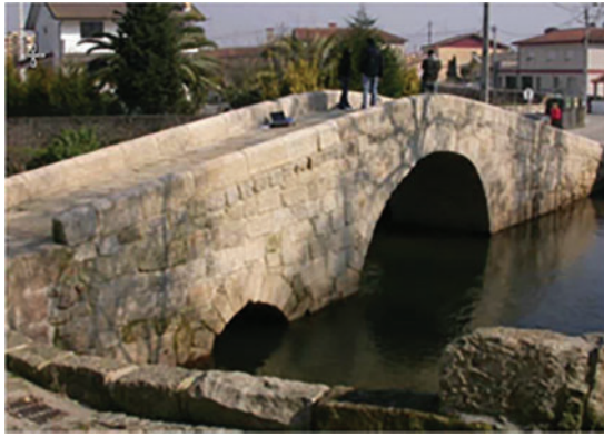
Figure 10. Examples of joint repointing on the Sao Lazaro bridge 5
