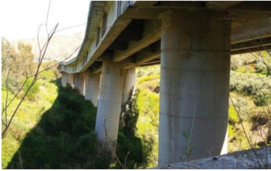
**Figure 7.** Examples of downslope pier rotation for the Himera Viaduct, Italy
