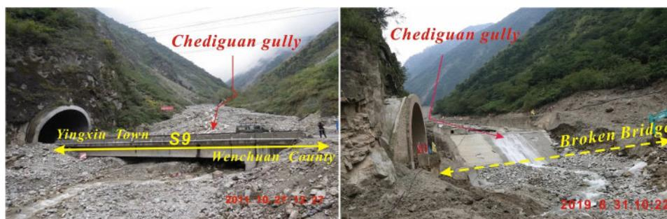
**Figure 10.** G213 Taiping Middle Bridge (China) after the first debris flow in 2011 and following its complete collapse in 2019<sup>35</sup>
