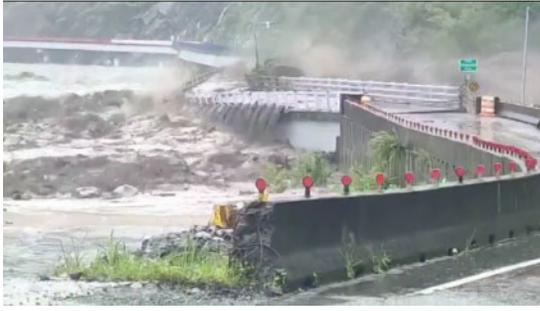
**Figure 9.** Minbaklu Bridge during the collapse caused by a mudflow on August 7, 2021
