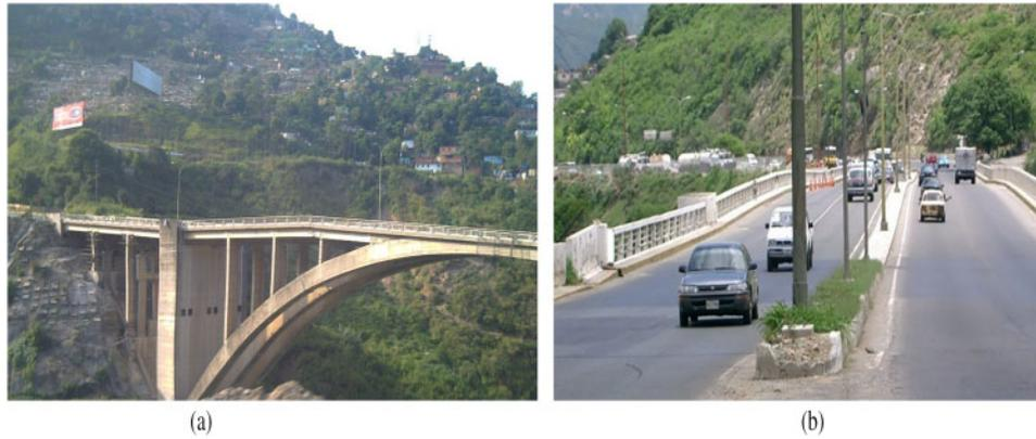
**Figure 4.** Lateral and frontal views of Viaduct 1 of Caracas–La Guaira (Venezuela) before its collapse on March 19, 2006, showing significant deck arching
