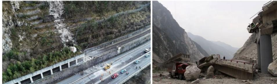
**Figure 12.** (a) The Pescatore Viaduct in Italy, impacted by falling rock blocks on January 12, 2024. (b) The Chediguan Bridge (China) collapsed following the impact with a boulder (July 25, 2009)
