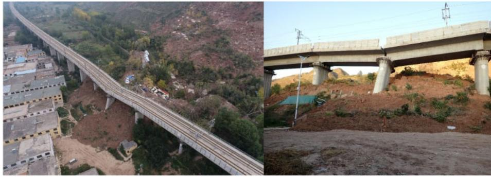
**Figure 11.** Landslide at the LX high-speed railway viaduct near Xining (China) on September 15, 2022 (courtesy of Ye Chen and Kongming Yan, adapted from Wang et al.<sup>36</sup>)
