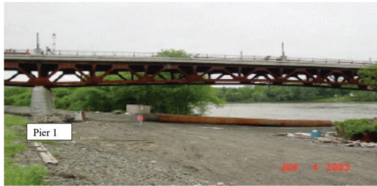
Figure 3. Span 2 downstream view
