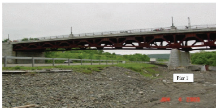
Figure 2. Span 1 downstream view
