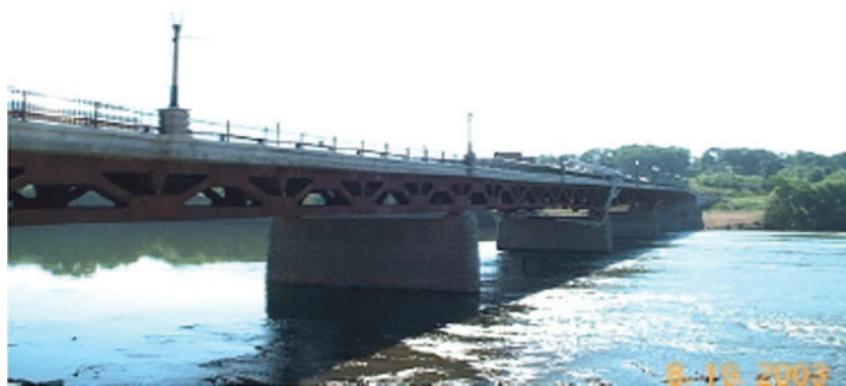
Figure 1. Court street bridge
