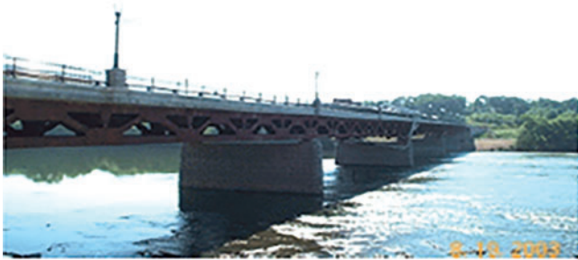
Figure 1. Court street bridge
