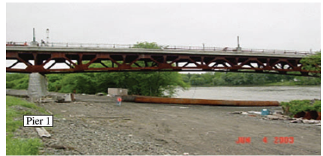
Figure 3. Span 2 downstream view
