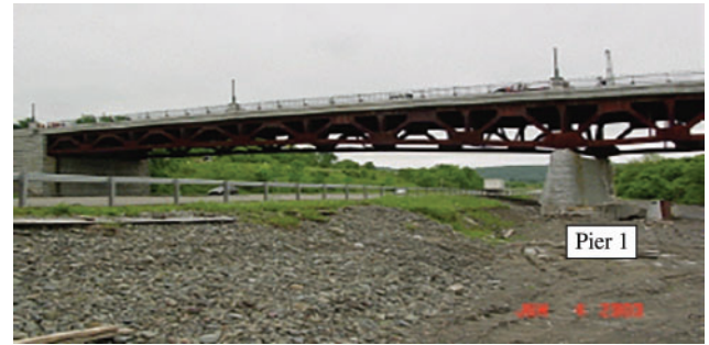
Figure 2. Span 1 downstream view
