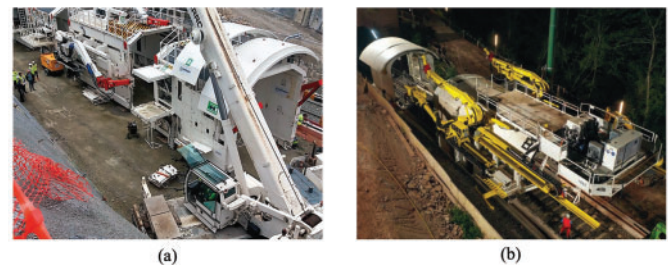
Figure 20. TEMs used for the (a) Gaintxurizqueta, Loyola, and Capuchinos tunnels 63 and (b) Kuckuckslay tunnel 12
